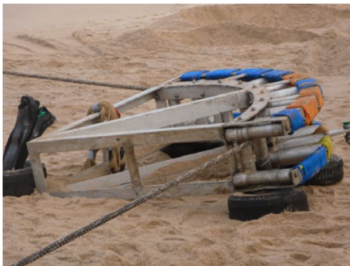
Quadrant used to pull the cable onshore
